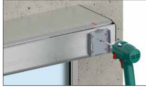
Alt kapak vidalanır. / Lower cover is screwed.
